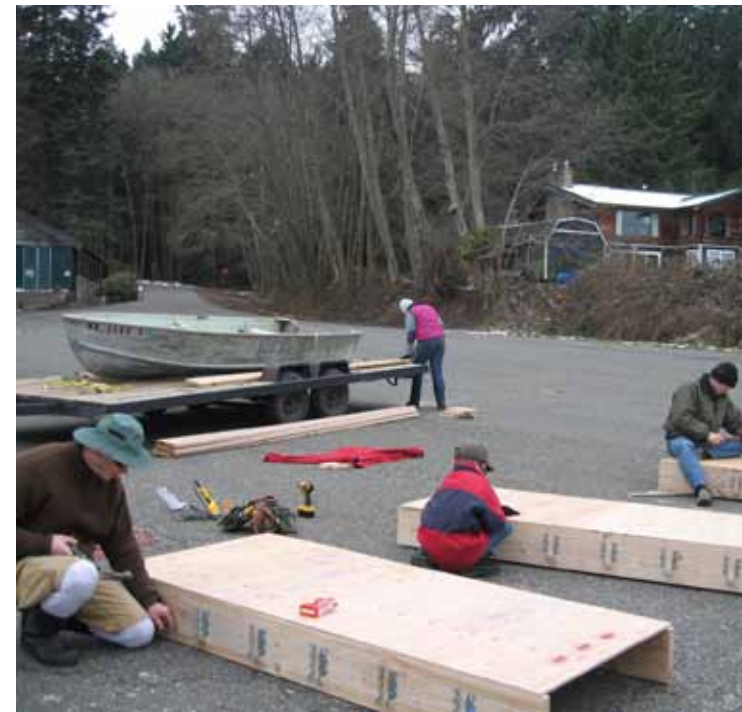
Volunteers help construct mussel float on Vashon Island.
